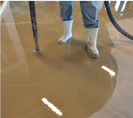
Figure 7.8 – Application of self-leveling underlayment over a primed concrete substrate.
