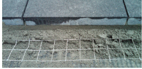
Figure 7.6 – Example of a non-bonded, wire-reinforced mortar bed. Wire mesh is placed in the middle of the mortar bed and lapped together to ensure continuity.
