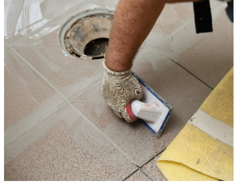
Figure 7.12 – Spreading of industrial epoxy grout.
