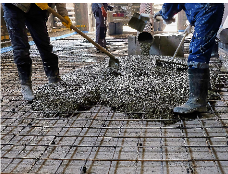
Figure 2.26 — Concrete pour over suspended composite steel pan floor construction.
