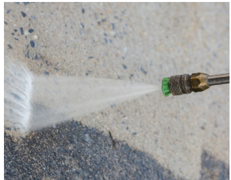
Figure 3.2 – High Pressure Water Washing.
