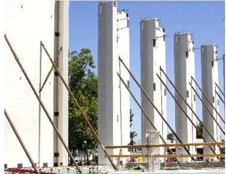
Figure 3.1 – Tilt-Up Concrete Panels erected into place.
