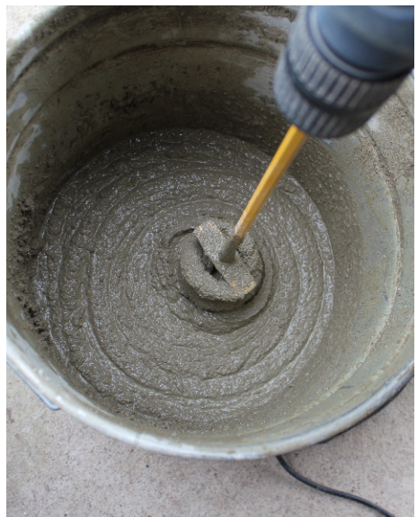
Figure 7.3 — Mixing of liquid latex-fortified portland cement thin-set mortar.
