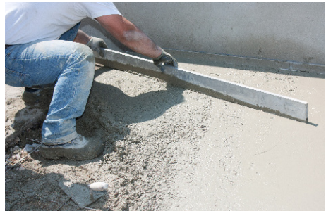
Figure 7.7 – Tile mechanic screeding a mortar bed.
