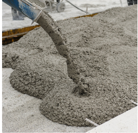
Figure 2.9 – Placement of Concrete Slab (Photo courtesy of California State DOT).
