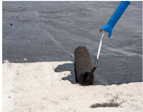
Figure 6.1 – Liquid applied membrane applied to concrete substrate.
